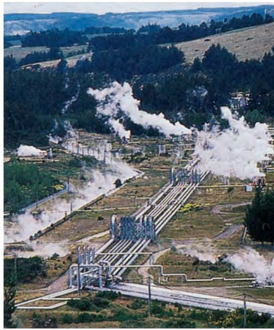
Power plant at Wairakei, New Zealand, that converts geothermal energy into electricity. (Jean-Pierre Horlin/The Image Bank.)
