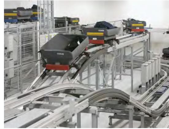
The speeds of the buggies transporting luggage between terminals at Heathrow International Airport are controlled by LIMs. (Vanderlande Industries.)
