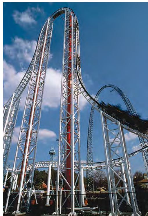
The Hypersonic XLC at Paramount's King's Dominion Amusement Park, Virginia, the world's first compressed-airlaunched roller coaster, goes from 0 to 80 miles per hour in 1.8 seconds. (Courtesy of King's Dominion Amusement Park.)
