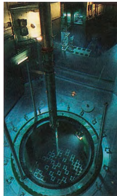
Control rods are inserted into this nuclear reactor at Tihange, Belgium. (Peter Miller/The Image Bank.)
