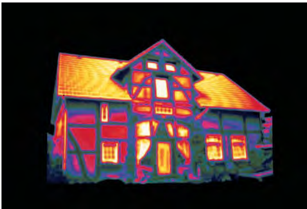
This thermogram of a house shows the heat being radiated to its surroundings. (Alfred Pasieka/Photo Researchers, Inc.)
