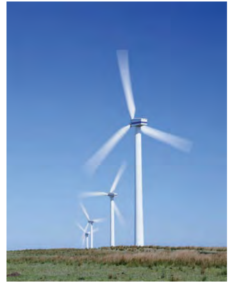
A wind farm converting the kinetic energy of the air to electrical energy. (Image Slate.)
