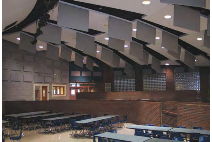
The baffles hanging from the ceiling and attached to the walls above the doorways are there to absorb sound. Their surfaces are made of acoustically dead material, like felt. (Courtesy of Perdue Acoustics.)
